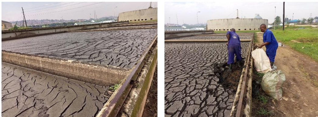
Figure 3. 2: Two (2) weeks old sewage sludge sample picking at Bugolobi STP.
