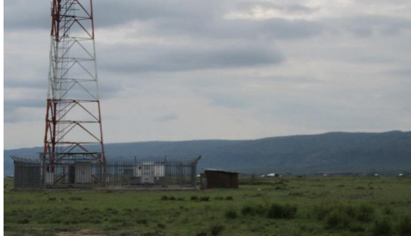
Plate B. 6 telecommunication tower in Tonya B
