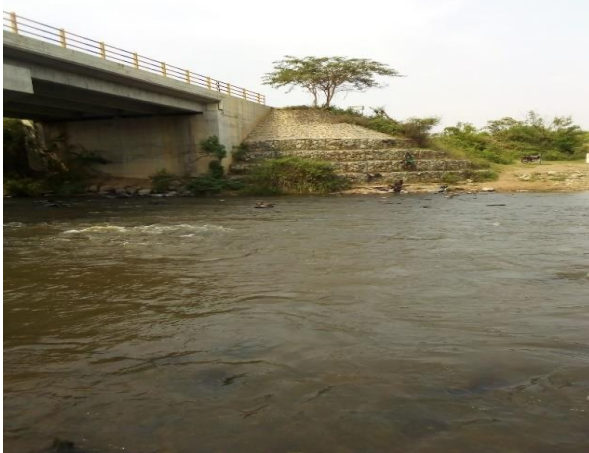
Plate B. 9 Wambabya bridge and Kaiso Tonya road
