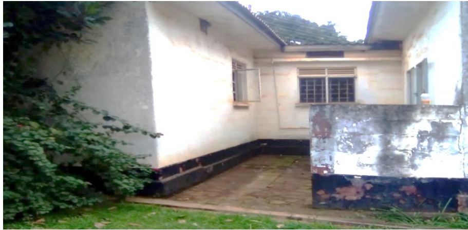
Figure 4. 3: Department of Performing Arts after renovation
