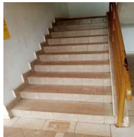
Photograph 9: Showing treads in a flight
