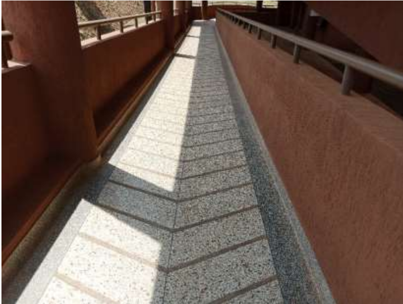
Photograph 10: Showing a well constructed ramp
