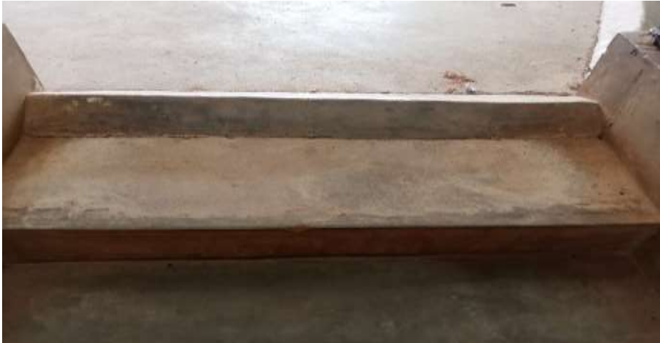
Photograph 5: Showing steps with a triangular barrier at the landing
