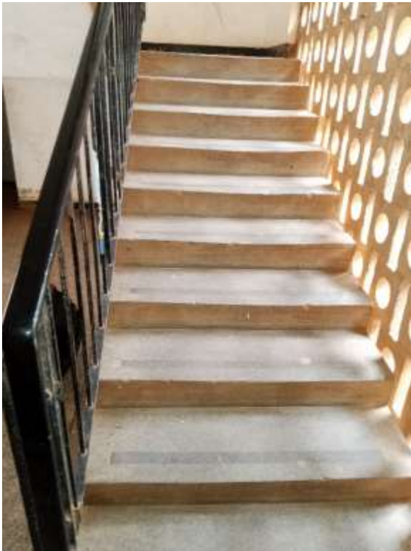
Photograph 11: Showing faded nosing contrast
