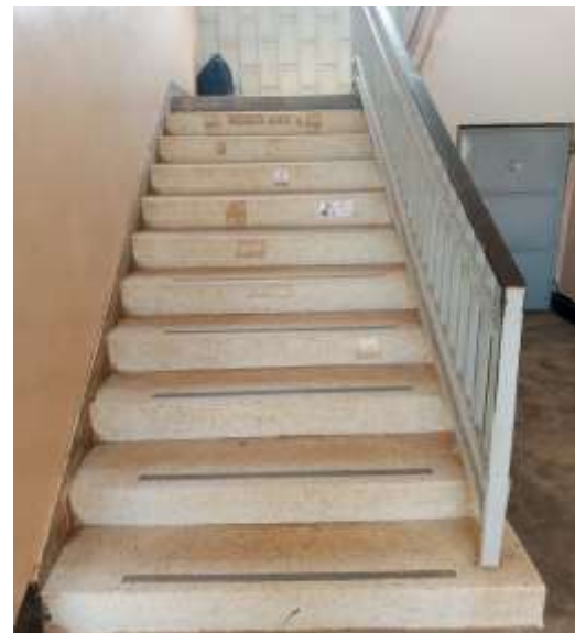
Photograph 4: Showing handrails on one side
