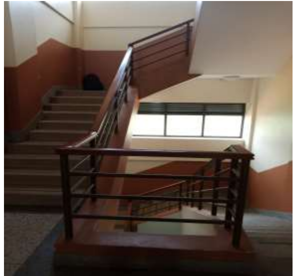
Photograph 2: Showing continuous handrail
