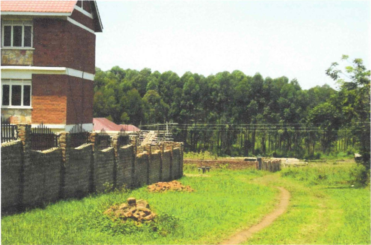
Figure 4.7: Building located near forest reserve in Maluku Ward in Industrial Division
