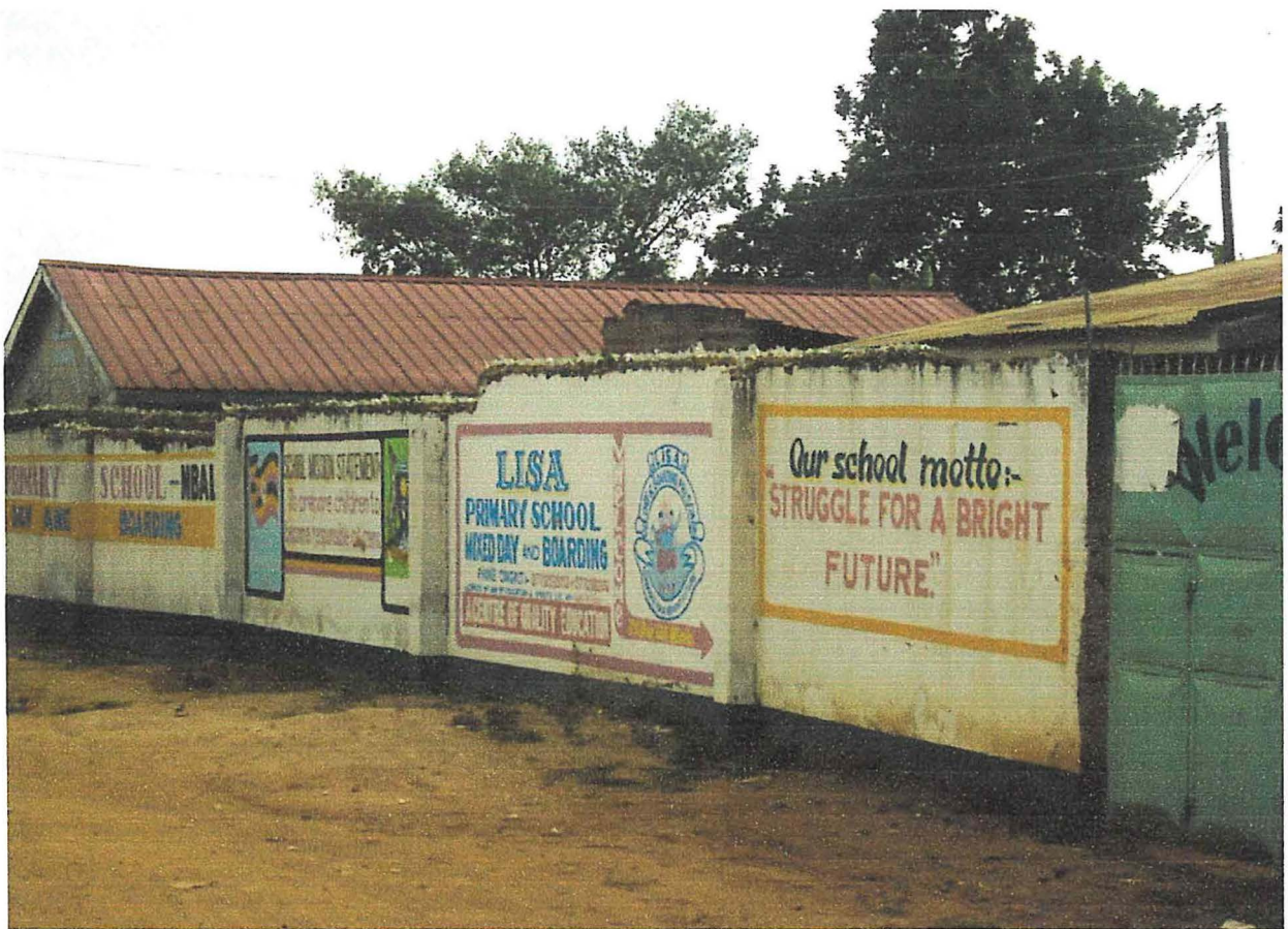
Figure 4.5: Former residential premises/structures that have been turned into a school in Namakwekwe Estate in Northern Division
