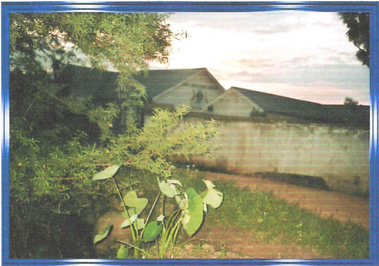
Figure 4.19: A school built in a wetland in southern part of Mbale Industrial Division
