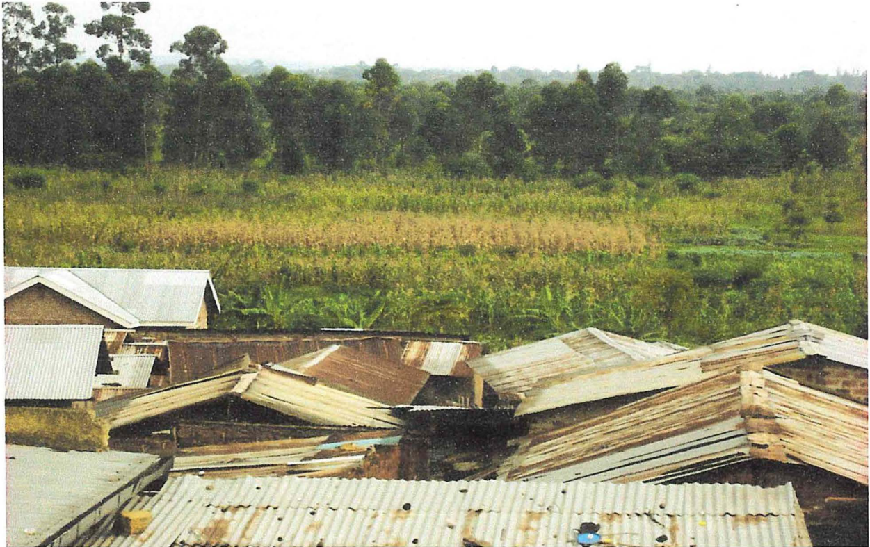
Figure 4.23: Unplanned settlements (Shaba Slums) in Maluku Ward in Industrial Division.
