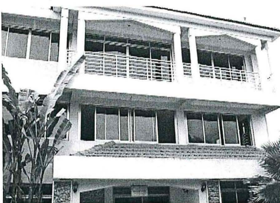
Front view upscale facility
