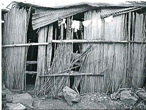
Front view lower scale facility
