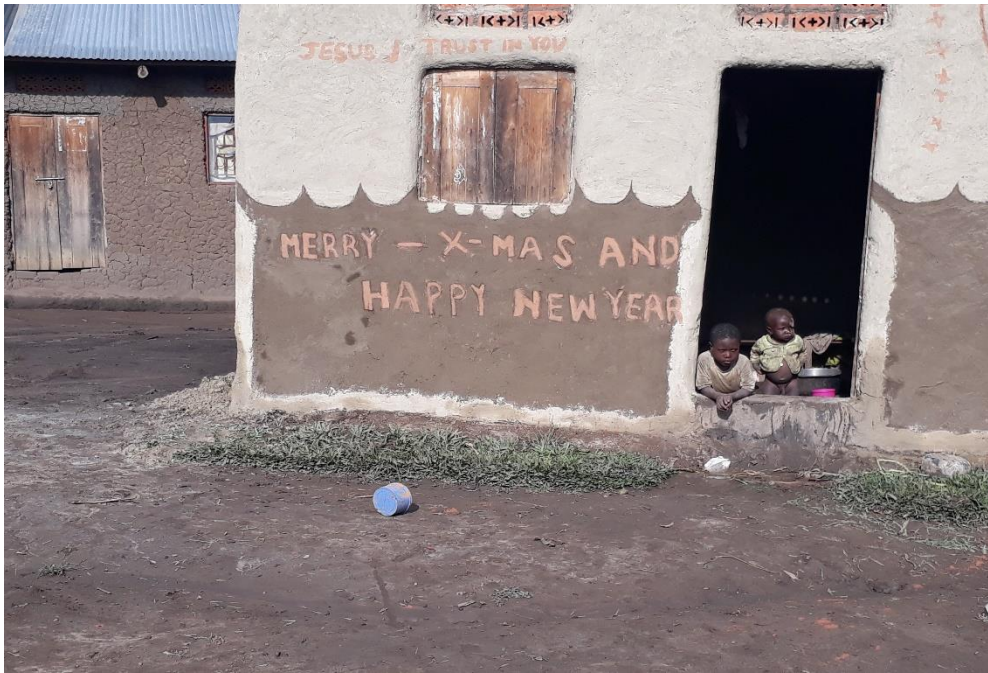
Figure 4. 10: Some of the buildings exposed to dam flood hazard in Kabuyanda flood plain
