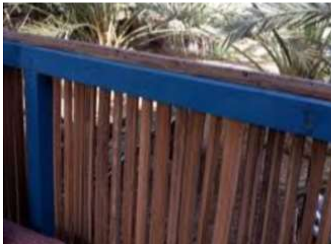
Figure 2.10: Fence made from date palm branches.
