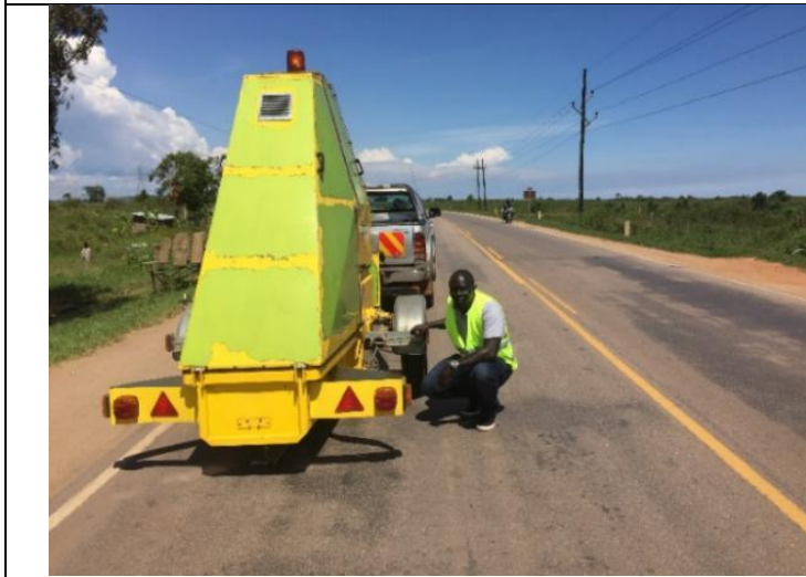
FWD testing at Km 98+210
